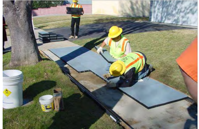
Workers installing rubber sidewalk pavers.
