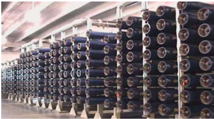
Figure XX. Membrane pressure vessels organized into treatment trains at the Sunrise, FL brackish water desalination plant (Image source: http://www.biwater.com/Images/content/1724/449510.jpg )
