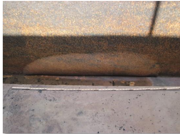
Photo 3-83. Approx. 54-inch-long by 12-inch-wide coating blister on north wall of south pass.
