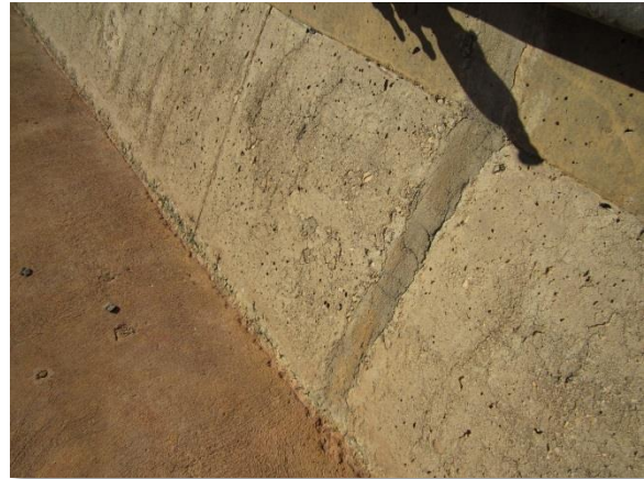
Photo A-53. Construction joints on west wall with deteriorating mortar overlay (typical).
