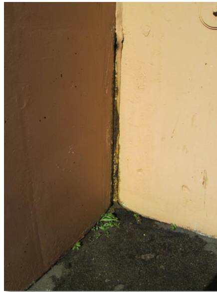
Photo C-12. Effluent tower separating from clarifier wall.
