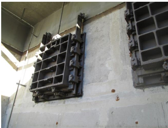
Photo A-11. Multiple small sources of corrosion staining on north wall.
