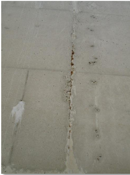
Photo A-9. Loss of mortar over construction joint on east wall about 350 feet south of north wall.
