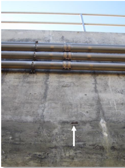
Photo A-60. Typical minor spalling on west wall.
