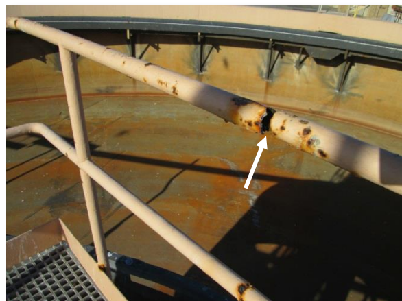
Photo 3-69. Corroded (separated) railing at end of PC 1 catwalk.
