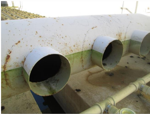
Photo 3-54. Steel manifold pipe with minor coating failure and corrosion.
