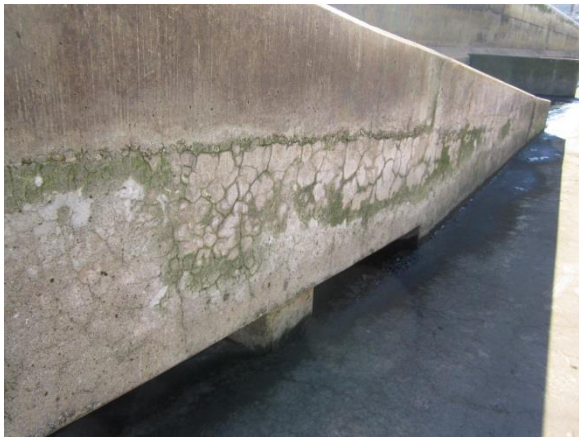
Photo 3-15. Cracked surface layer near bottom of ramp.
