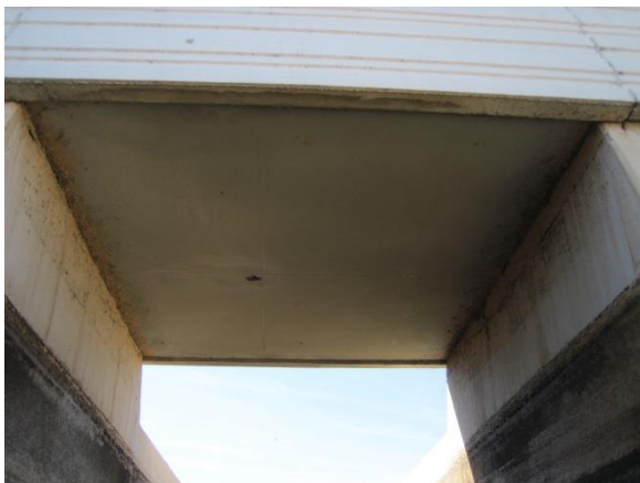
Photo 3-76. No cracks or spalls were observed on the underside of the pedestrian bridge.
