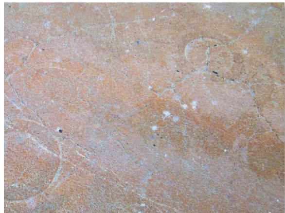
Photo A-24. Typical cracks in PC 1 floor.
