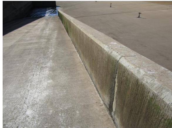
Photo 3-17. Cracks in a few locations are visible on both sides of the wall and appear to extend through it.
