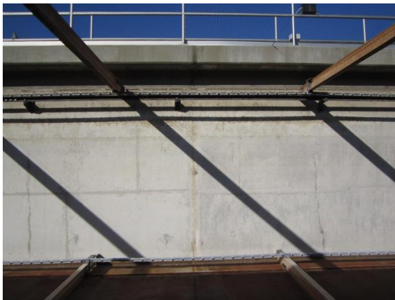
Photo A-39. Evidence of possible seepage through construction joint near midpoint of north wall (south wall similar).
