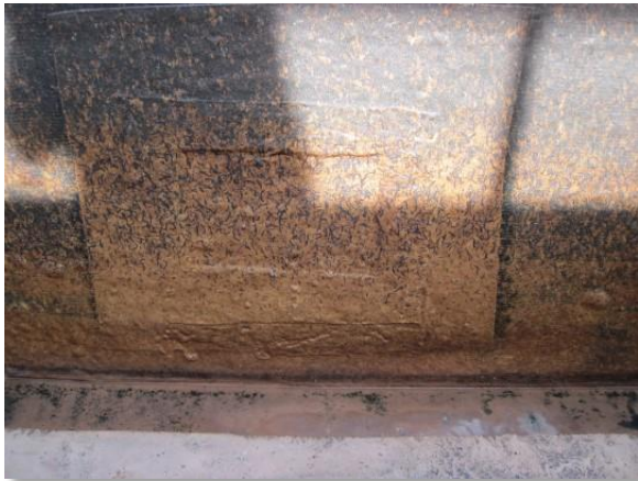
Photo 3-82. Approx. 24-inch-long by 24-inch-wide coating repair section. This section is hollow, which suggests the coating is not properly adhered.
