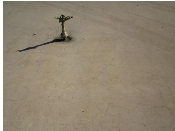
Photo 3-4. Typical cracking on West FEB floor.
