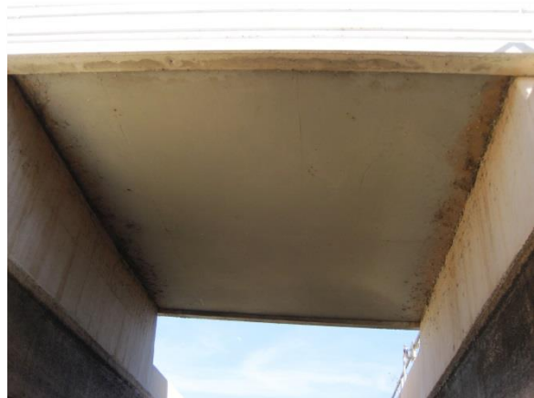
Photo 3-81. No cracks or spalls were observed on the underside of the pedestrian bridge.
