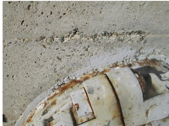
Photo A-14. Rock pocket above manifold pipe penetration about 305 feet south of north wall.
