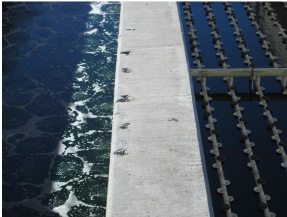
Photo 3-46. Exposed ends of reinforcing bars at top of wall between ASTs 1B and 1C.
