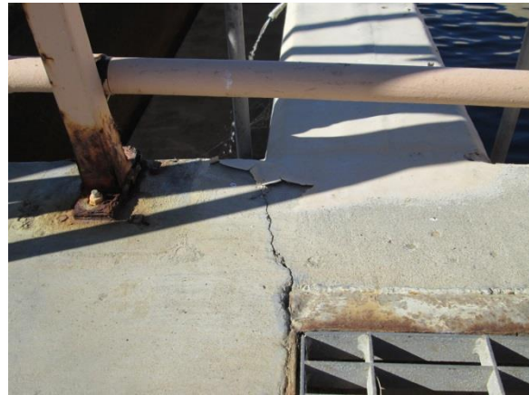
Photo 3-75. Crack observed on the deck level at the northeast corner of the north pass.
