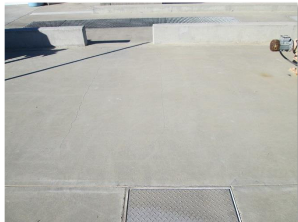
Photo C-26. Cracking in slab over west end of basin (more extensive than SST 2).
