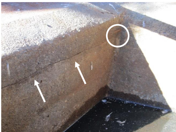
Photo 3-62. Grout or mortar joint at the center sludge pit. A short section of apparently exposed reinforcing steel was also visible (circle).
