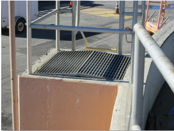
Photo C-11. Grating on top of effluent tower not seated properly, reportedly due to corrosion products.
