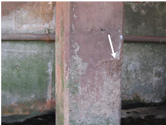
Photo 3-26. Damaged corner on column.
