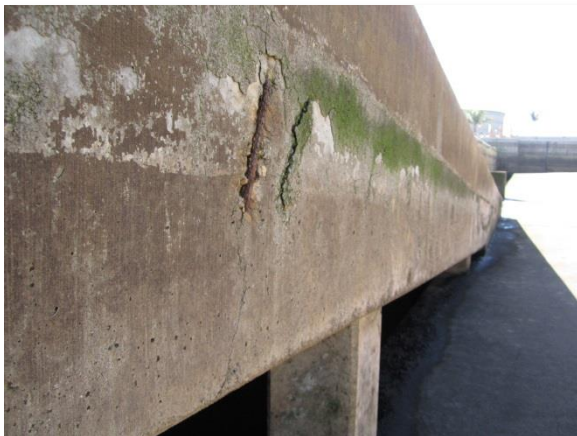
Photo 3-18. Typical minor spalling on outside of ramp.
