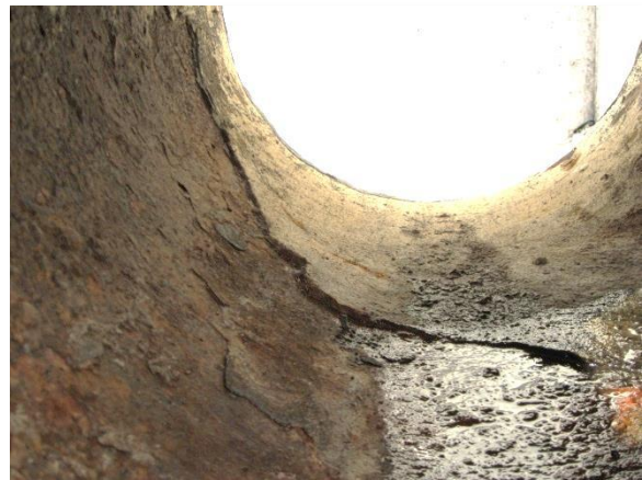
Photo A-47. Damage to cement mortar lining inside inlet tee at east wall.
