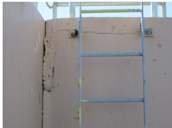
Photo C-16. Broken concrete at top of effluent tower.
