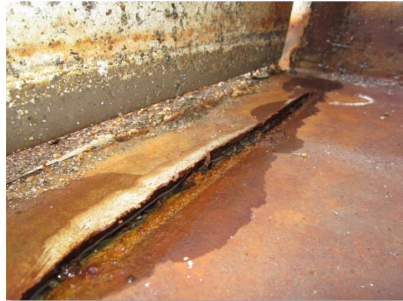
Photo 3-37. Deteriorated sealant at expansion joint near west end of SST 2 with evidence of possible infiltration.
