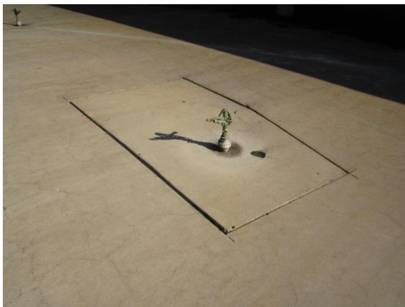
Photo 3-22. Joints surrounding sprinkler near north end of FEB.
