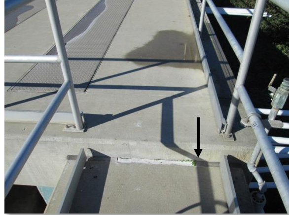
Photo C-35. Weeds growing from expansion joints.
