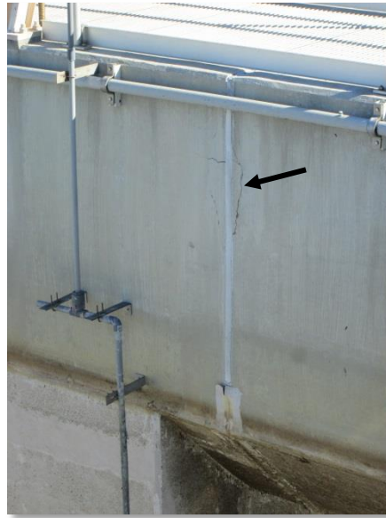
Photo C-8. Spalling concrete adjacent to expansion joint.
