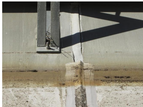
Photo A-12. Typical sealant in expansion joint with shrinkage and gaps.
