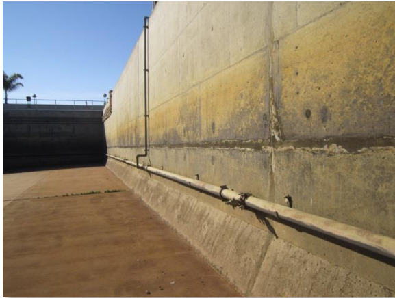
Photo A-52. Construction joints on west wall with deteriorating mortar overlay (typical).
