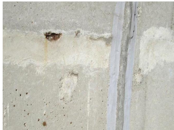
Photo 3-45. Spalling mortar with moderate corrosion of reinforcing steel near expansion joint 396 feet south of north wall.
