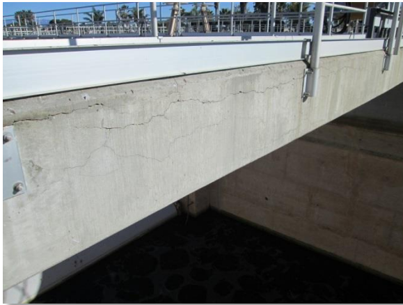
Photo C-1. Cracking on edge of walkway.
