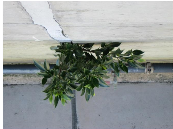
Photo C-24. Weeds growing from sealant in east wall.
