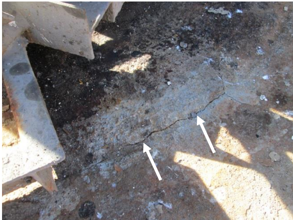
Photo A-25. Cracks near center column have separated about 1/8 of an inch.
