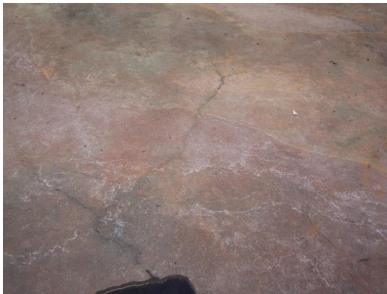
Photo 3-35. Typical minor cracking on floor of SST 2. Possible infiltration visible at bottom of image.
