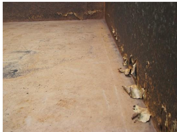
Photo 3-77. Detail of coating overspray on the floor and coating delamination.
