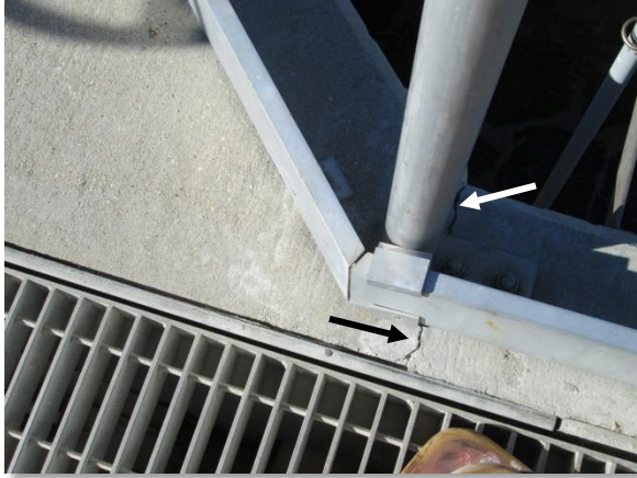
Photo C-7. Cracking at southeast corner of basin.
