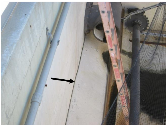
Photo 3-38. Gap between east wall and fill concrete.
