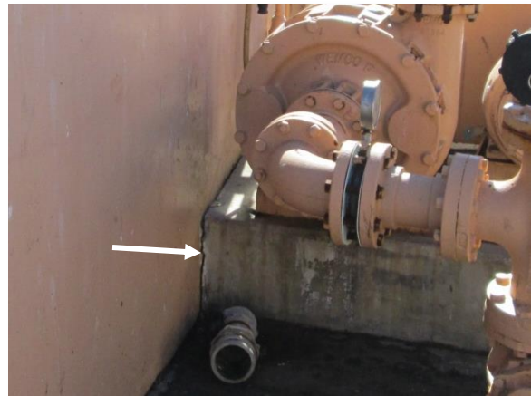
Photo A-28. Gap between pump base and clarifier wall.
