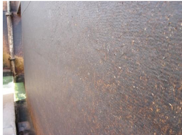
Photo 3-73. Area of hollow coating on south wall of north pass suggests the coating is not properly adhered.
