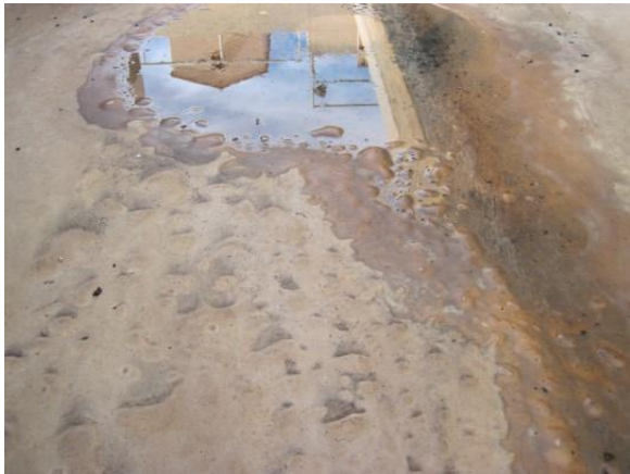
Photo 3-78. Blisters on floor were observed along a 40-foot-long section of the floor.
