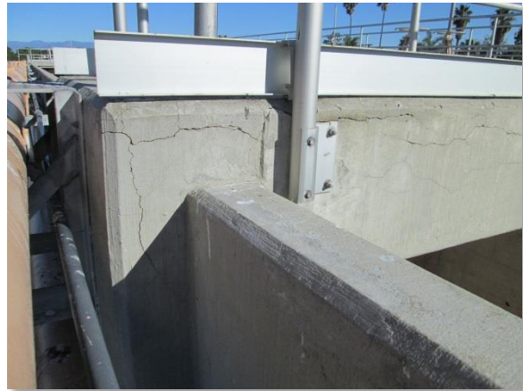
Photo C-2. Cracking on edge of walkway.
