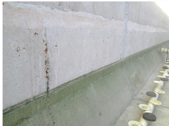
Photo 3-49. Exposed steel (possible vertical reinforcing bar) about 4 feet above floor on west wall and about 95 feet south of north wall.
