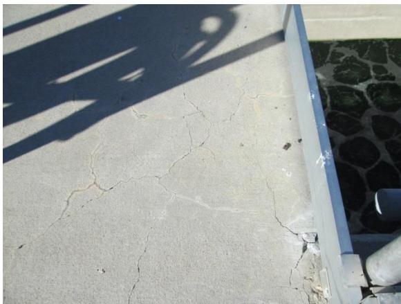
Photo C-5. Cracking on top surface of walkway.
