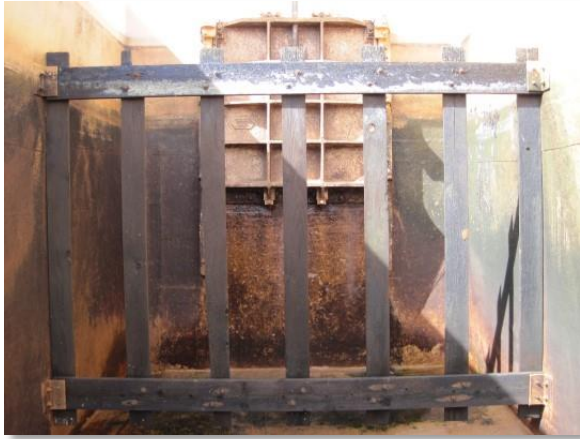
Photo 3-70. The bolts and supports of the baffles were in VANDA Level 1 condition.
