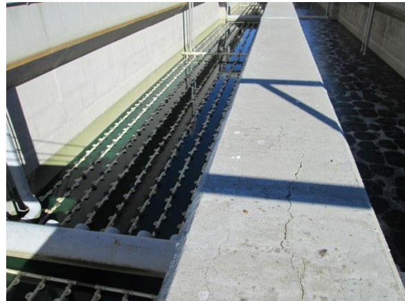
Photo 3-47. Cracking on top surface of wall between ASTs 1B and 1C (typical).
