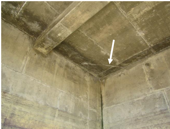
Photo A-62. Minor cracking and efflorescence on bottom of platform at northwest corner of West FEB.
