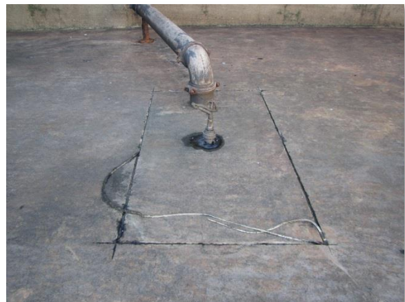
Photo 3-23. Joints around sprinkler near south end of FEB, with sealant coming loose.
