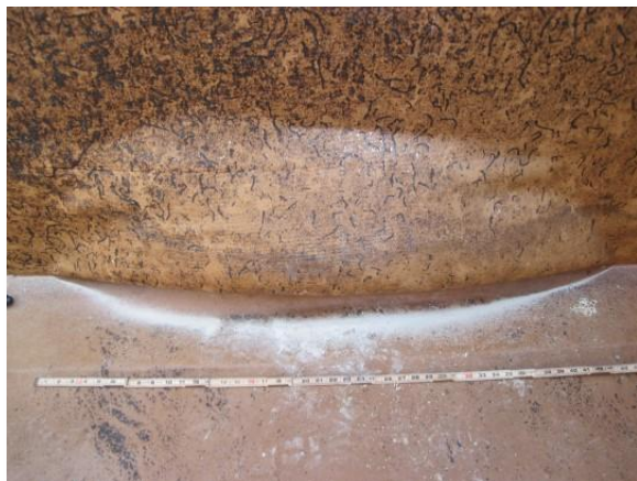
Photo 3-84. Approx. 48-inch-long by 18-inch-wide blister at east end of south pass on outside east wall of CCC.
