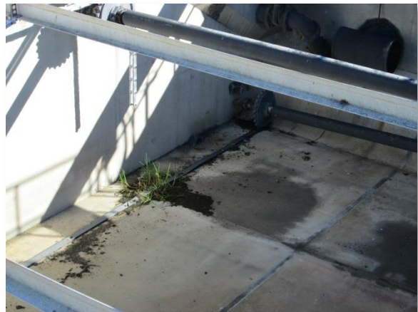
Photo C-33. Weeds growing from expansion joints.
