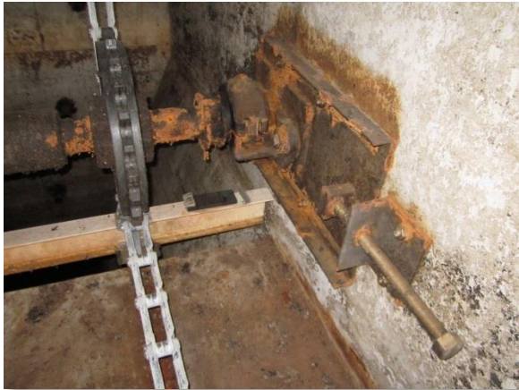
Photo A-44. Coating failure and minor corrosion on brackets for skimmer system.
