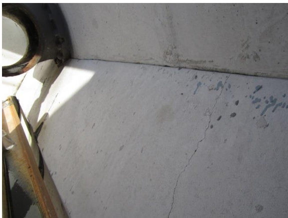
Photo A-43. Minor cracking in tapered fill concrete at east wall of SST 2.
