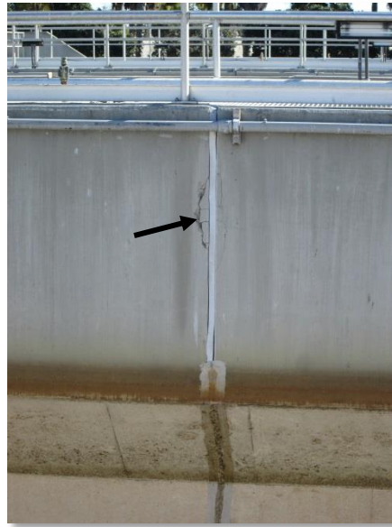
Photo C-4. Spalling concrete adjacent to expansion joint.
