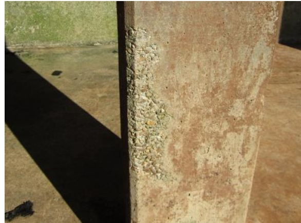
Photo 3-25. Typical exposed aggregate on column.
