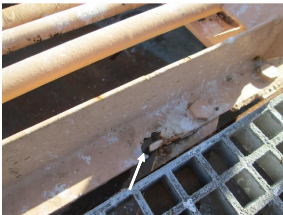
Photo 3-68. Holes through lower members of catwalk truss. Corrosion damage has been painted over.
