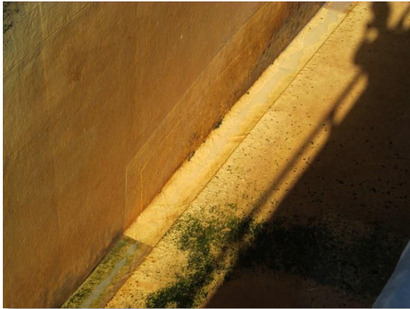
Photo A-75. Typical coating patch.
