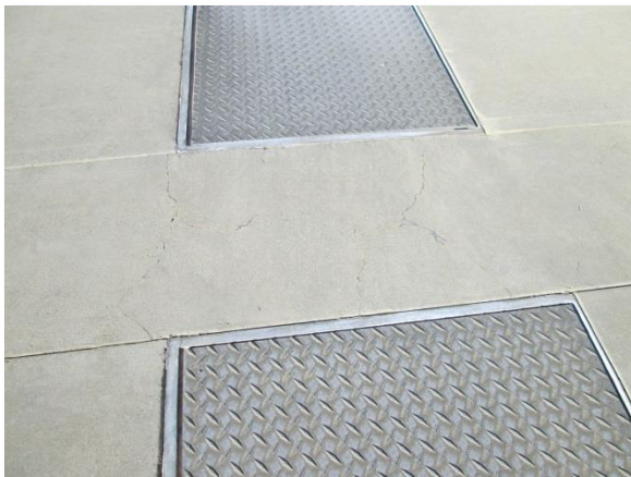
Photo C-25. Cracking in slab over west end of basin.
