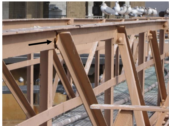
Photo A-32. Loose bracing on PC 1 catwalk truss due to broken or corroded welds.
