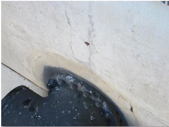
Photo C-27. Cracking in east wall above inlet tee.
