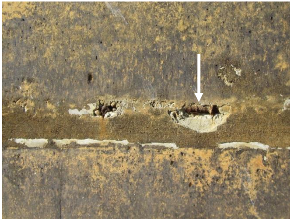
Photo 3-5. Broken mortar and exposed reinforcing bar at some locations along construction joint in west wall.
