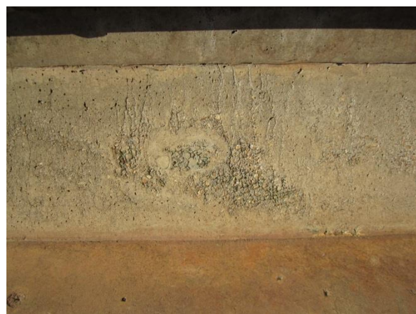
Photo 3-12. Typical concrete surfaces along toe of west wall with intermittent areas of exposed aggregate.
