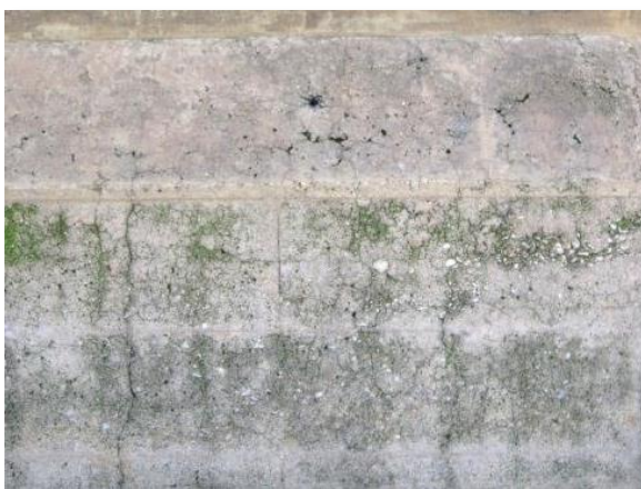
Photo 3-11. Bug holes and exposed aggregate along lower east wall.
