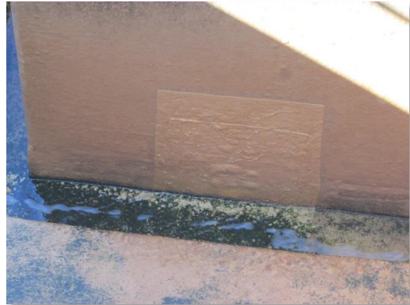
Photo A-76. Typical coating patch.
