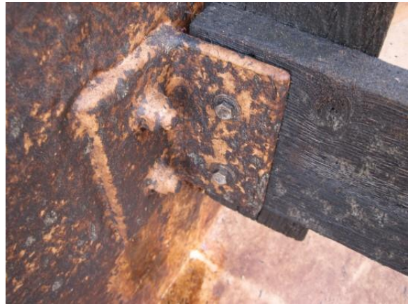
Photo 3-79. The coating on the brackets for the wooden baffles is in good condition.
