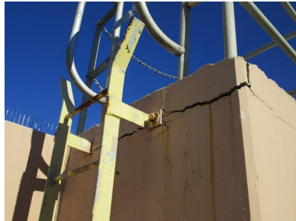
Photo C-10. Broken concrete at top of effluent tower.
