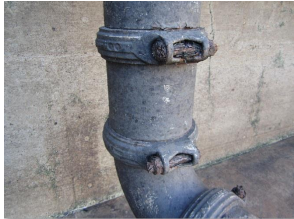
Photo A-65. Corroded hardware on Victaulic couplings for pipe at south wall.
