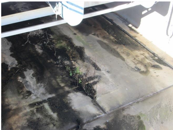
Photo C-32. Weeds growing from expansion joints.
