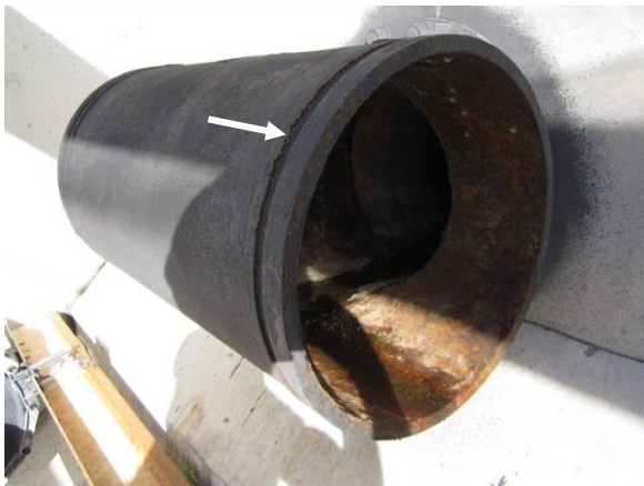
Photo A-46. Inlet tee at east wall. Arrow denotes minor coating failure and surface corrosion.
