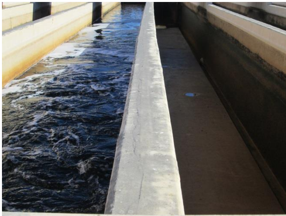
Photo A-74. Coating condition at top of north wall of north pass (North CCC at left).
