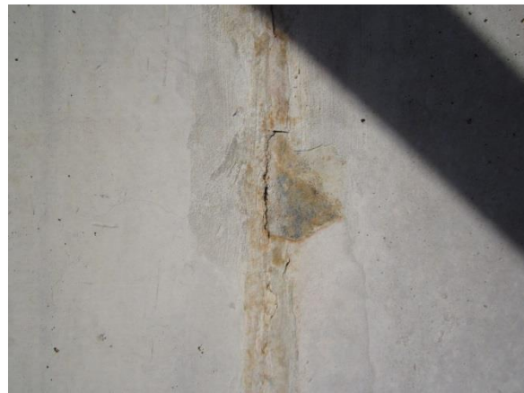
Photo A-40. Detail of possible seepage through construction joint near midpoint of north wall.
