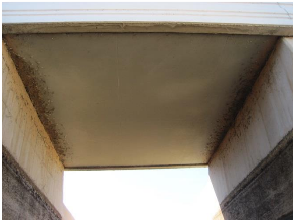
Photo 3-74. No cracks or spalls were observed on the underside of the pedestrian bridge.
