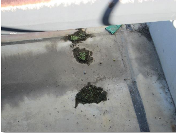
Photo C-34. Weeds growing from expansion joints.
