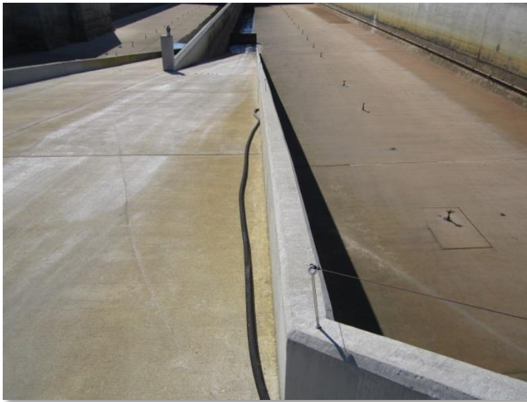
Photo 3-28. North end of wall along ramp. Low height of wall presents a fall hazard.
