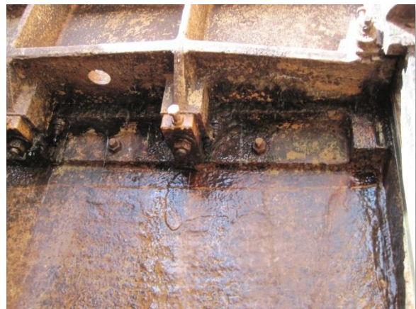
Photo 3-89. Minor leaking of the inlet sluice gate.
