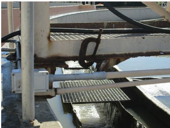
Photo C-17. Apparent broken welds on catwalk.
