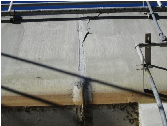
Photo 3-52. Spalling concrete adjacent to expansion joint on west wall about 303 feet south of north wall.
