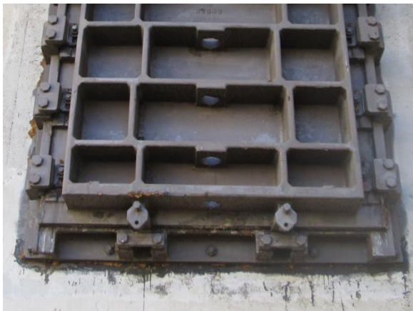
Photo A-15. Minor coating failure and corrosion on sluice gates and frames.
