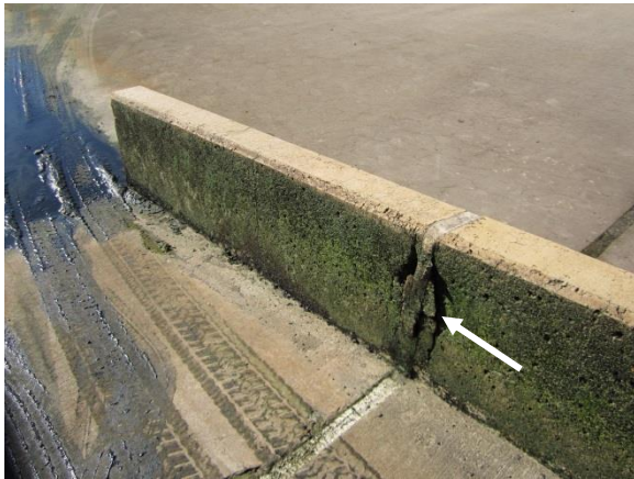
Photo 3-9. Spalled concrete adjacent to expansion joint in wall at bottom of ramp.
