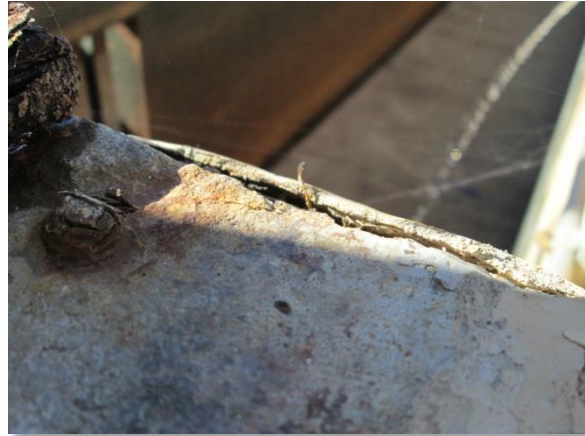
Photo A-80. Coating delamination at northeast corner.
