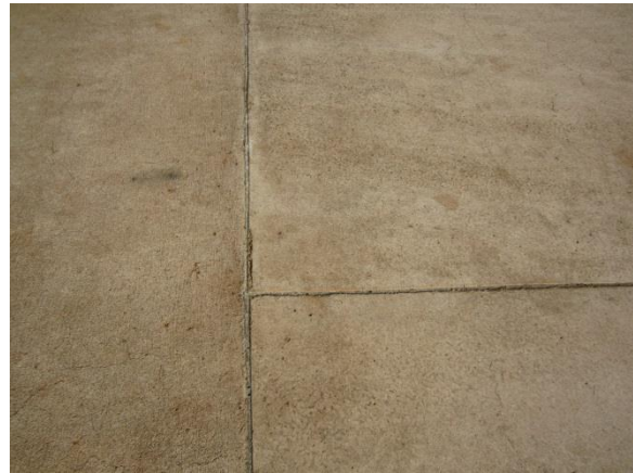
Photo 3-10. Typical control joints in floor.
