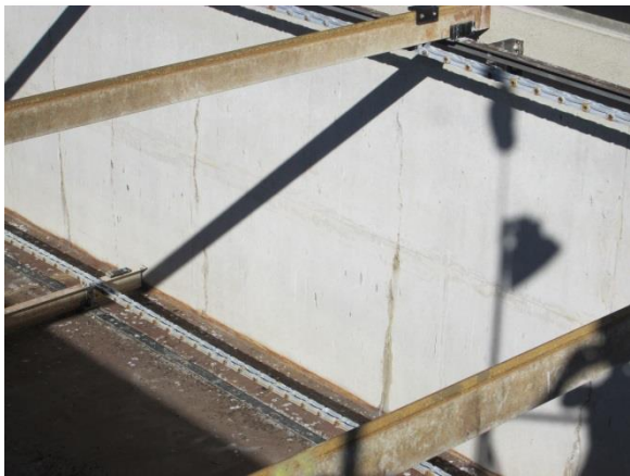
Photo C-28. Vertical cracks every few feet along length of north wall (similar to SST 2).
