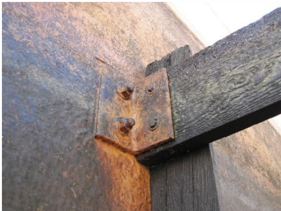
Photo 3-80. The coating on the brackets for the wooden baffles is in good condition.
