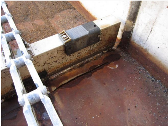
Photo 3-36. Deteriorated sealant at expansion joint near west end of SST 2 with evidence of possible infiltration.
