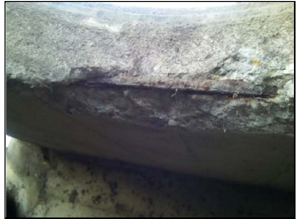
Exposed reinforcing steel
