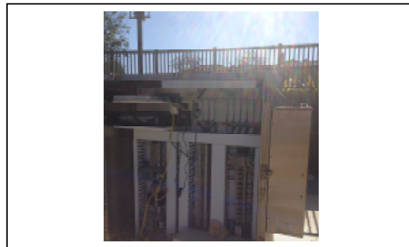
Picture – Panel Internal
