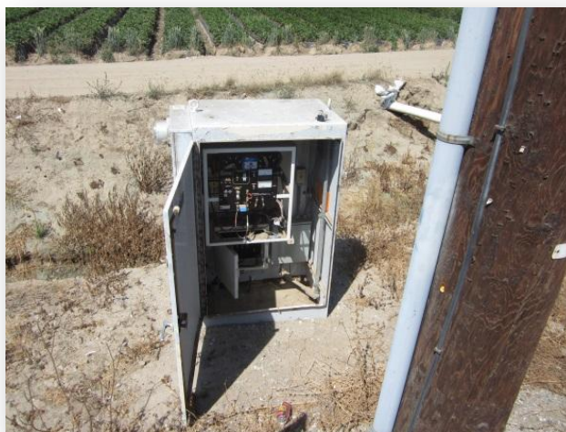
Photo 2) Cathodic Protection Rectifier on Del Norte Pipeline
