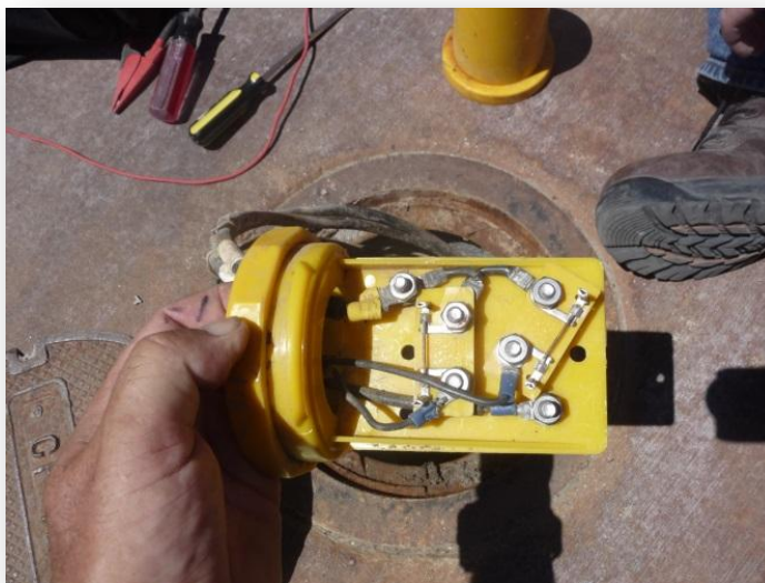
Photo 9) Cathodic Protection Anode Test Station at Water Treatment Plant
