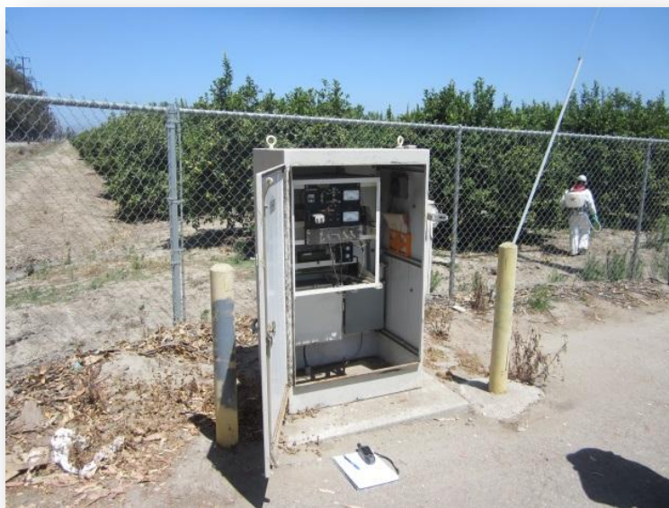
Photo 3) Cathodic Protection Rectifier #9 on Del Norte Pipeline
