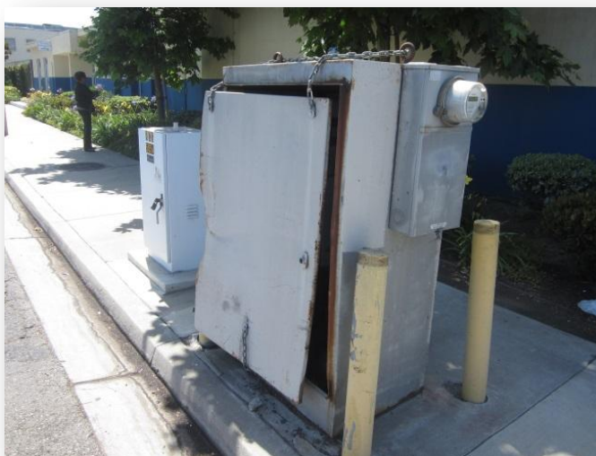
Photo 6) Cathodic Protection Rectifier on 3 rd Street Lateral. Rectifier and Anode Ground-Bed have Failed and Require Replacement.
