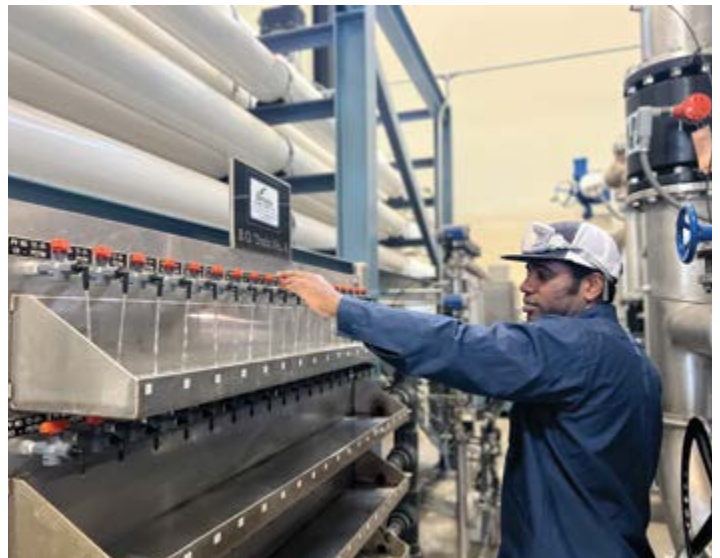
Operation staff testing the Desalter Facility membranes
