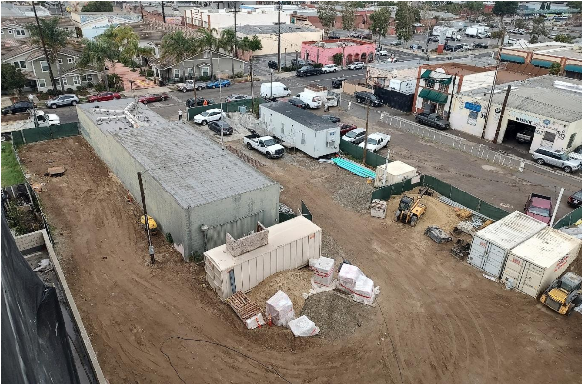
Figure 15 536 and 538 Meta Street Property Overview, Facing Northwest
