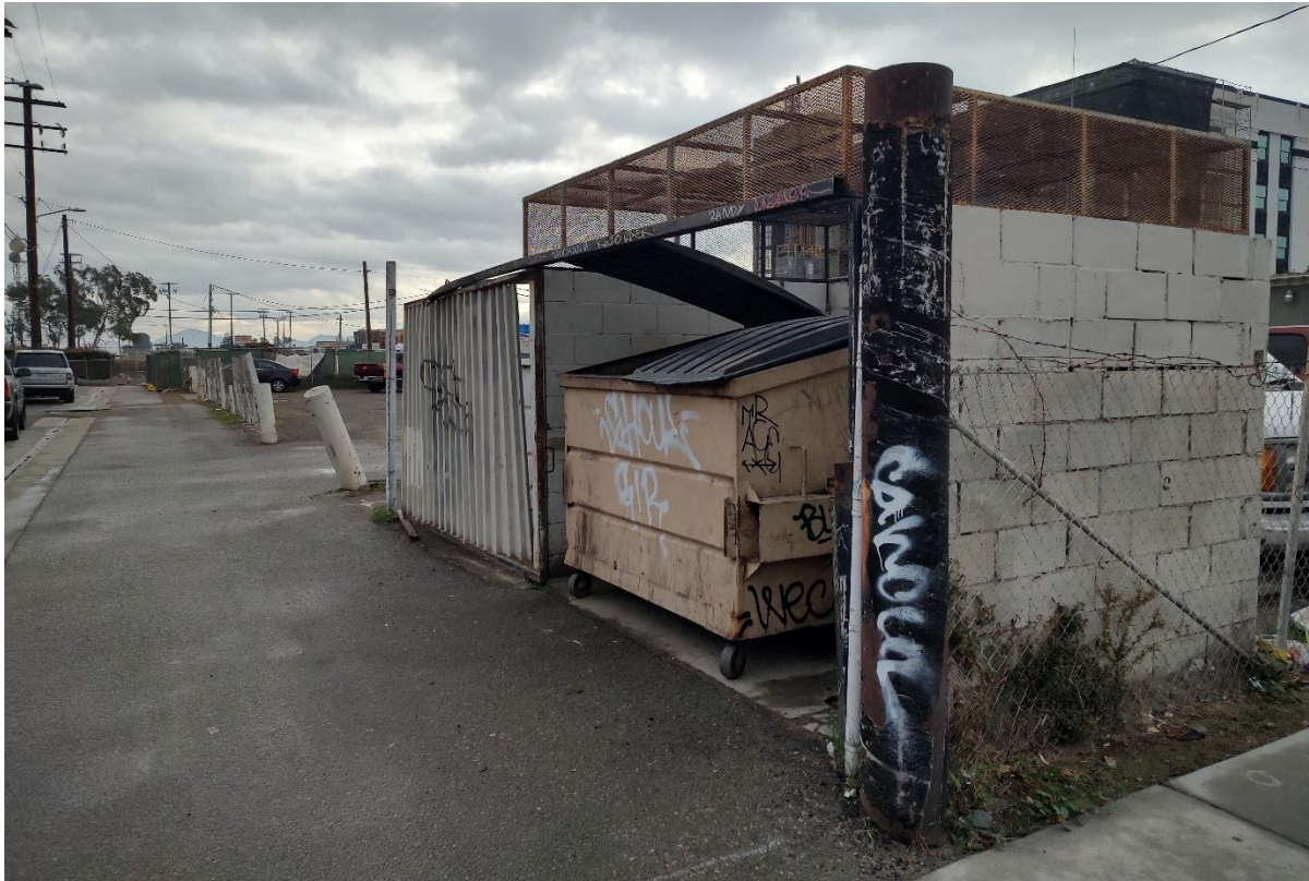
Figure 18 536 and 538 Meta Street South Trash Enclosure, Camera Facing Southeast
