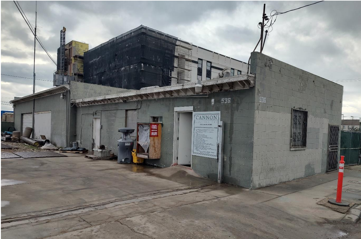
Figure 16 536 and 538 Meta Street North and West Elevations, Facing Southeast
