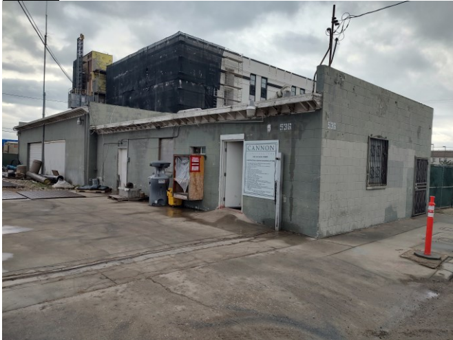
Photo 1: 536-538 Meta Street, North and West Elevations, View Southeast
