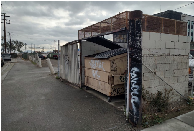
Photo 3: 536 and 538 Meta Street South Trash Enclosure, View Southeast
