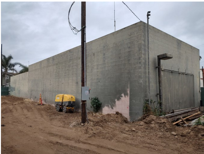
Photo 2: 536-538 Meta Street, South and East Elevations, View Northwest
