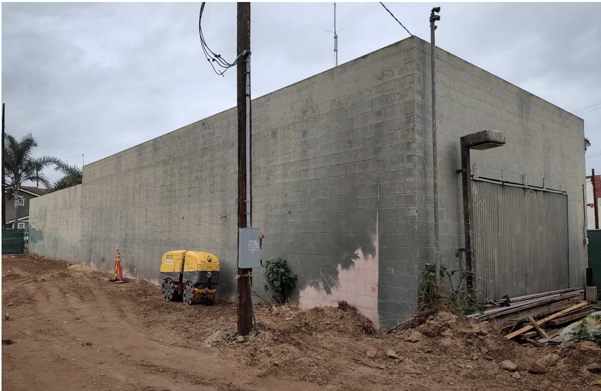
Figure 17 536 and 538 Meta Street South and East Elevations, Camera Facing Northwest
