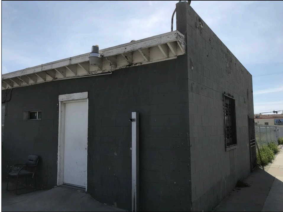
Photo 2: Western view of the subject building.
