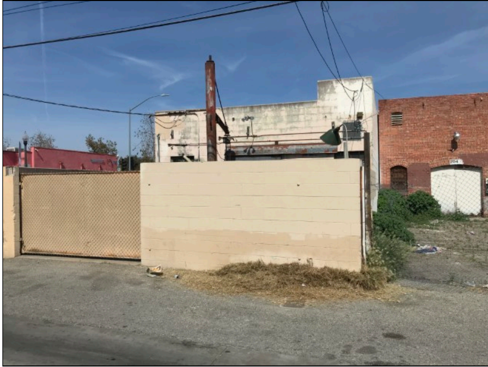
Photo 21: View of adjacent property to the north.
