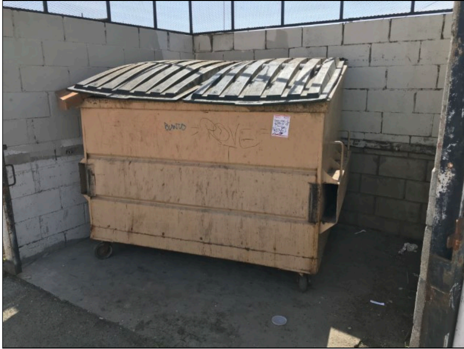
Photo 17: View of trash enclosure with a dumpster.
