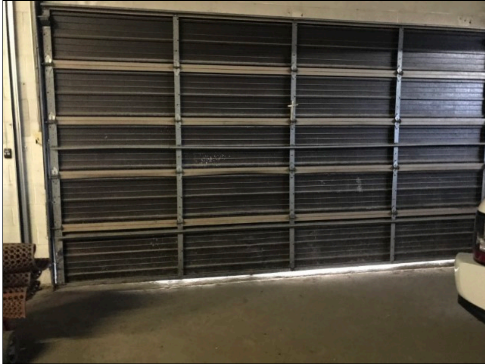
Photo 12: View of roll-up door for the warehouse.
