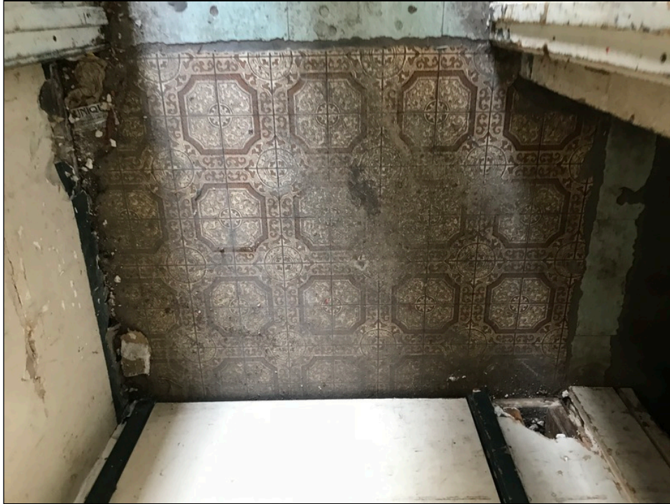
Photo 8: View of interior flooring.
