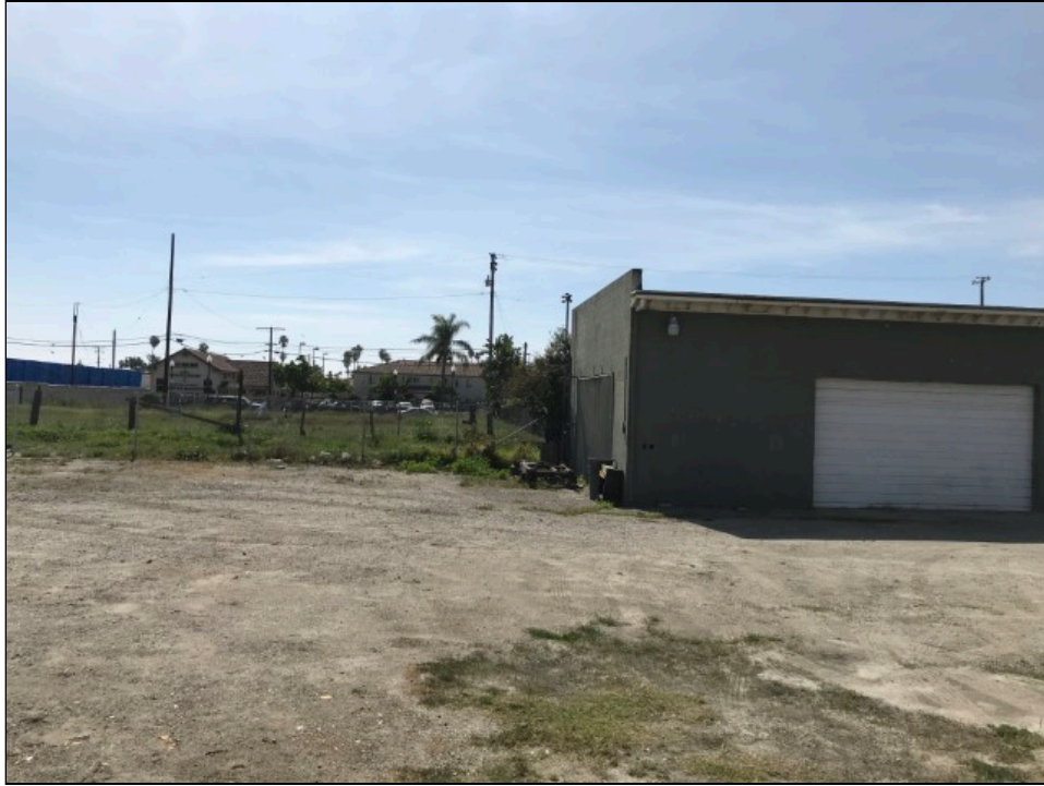
Photo 3: View of east side of subject building.
