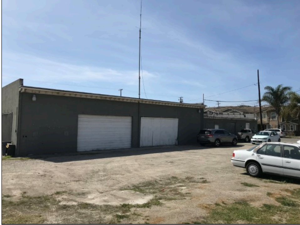
Photo 1: View of subject building looking south.
